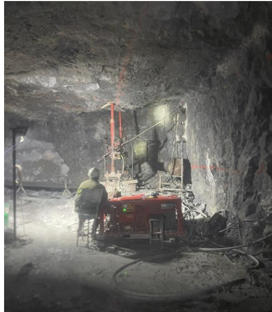
Figure 1: Underground drilling at #3 shaft
