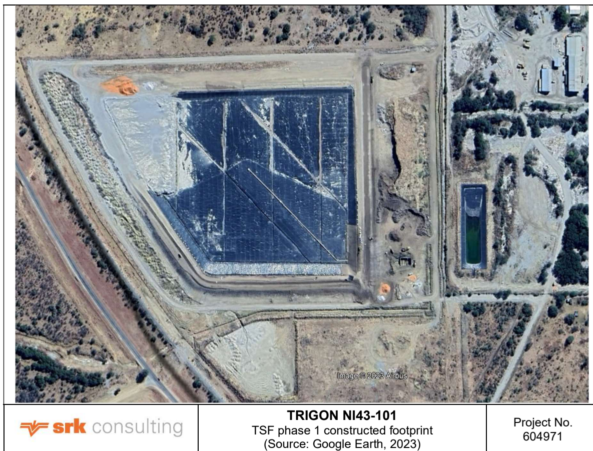
Figure 18-5: TSF Phase 1 Constructed Footprint
