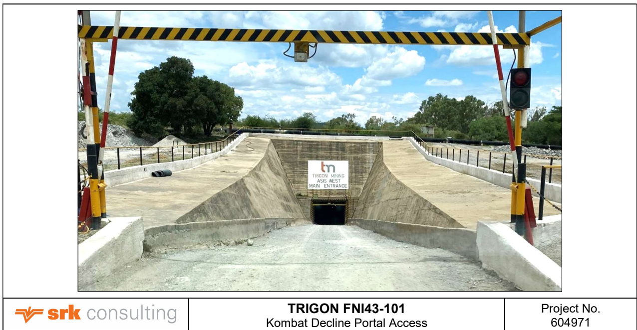
Figure 16-4: Decline Portal at Kombat Mine
